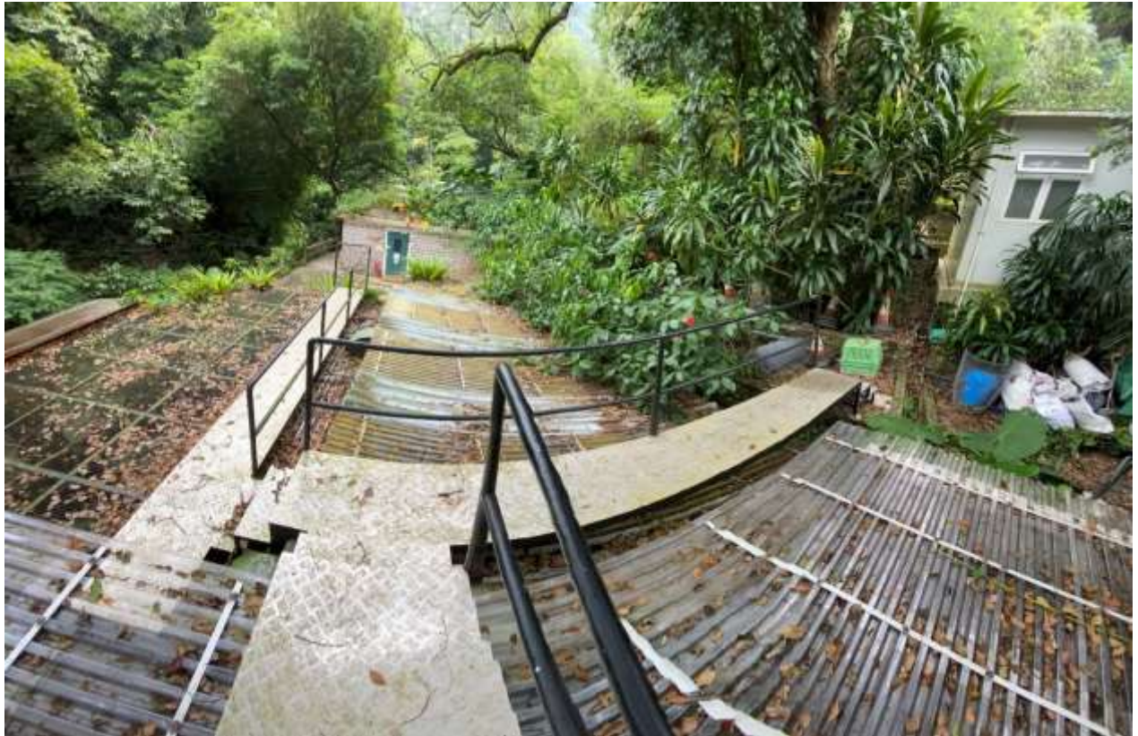
Fig. 21. Roof walks and railings allow safe access to facilities for cleaning and maintenance work
